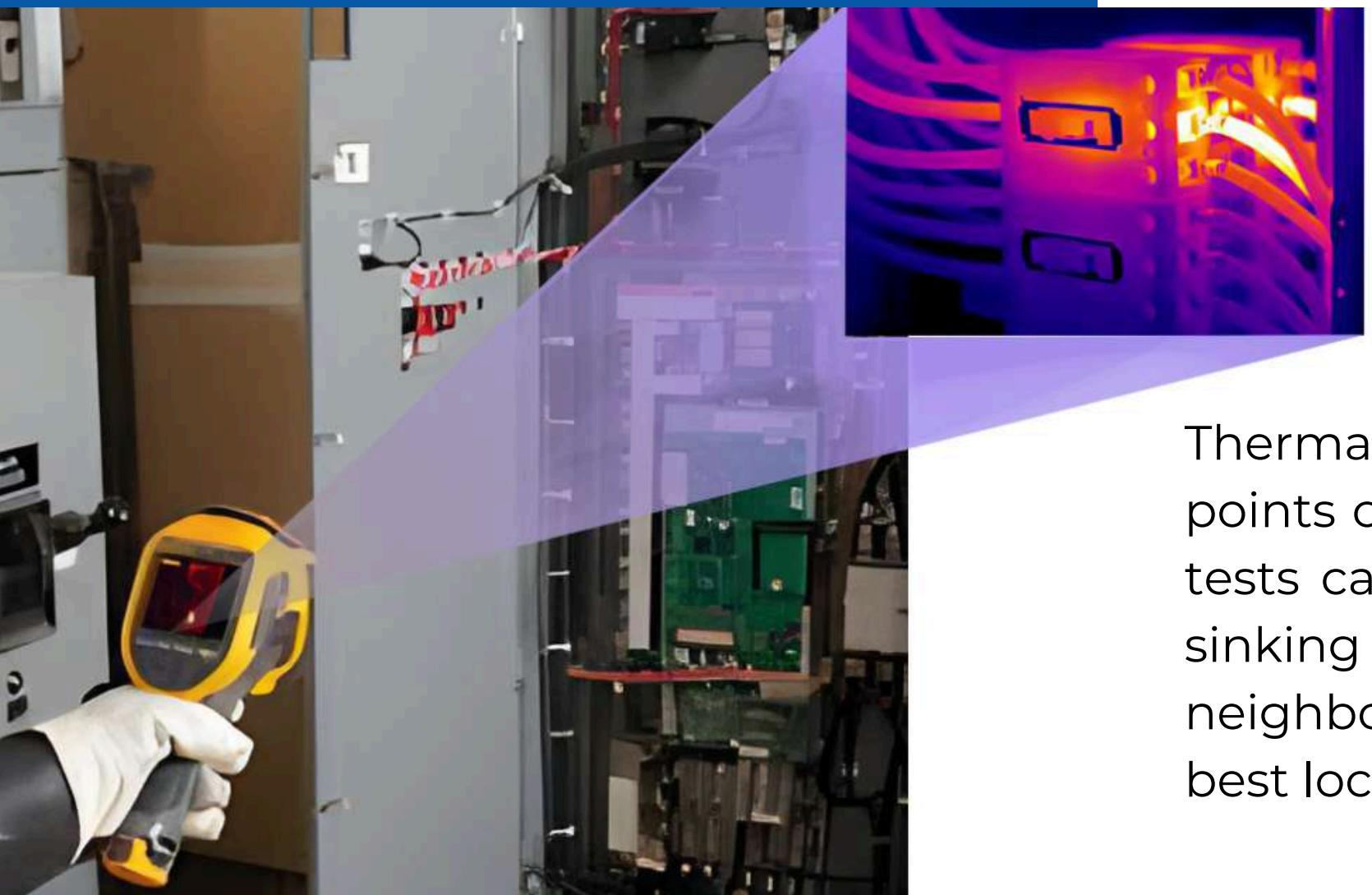
Using thermography, it is possible to check active installations and rapidly identify critical situations affecting energy distribution and electrical components (loose or corroded connections, load imbalance, overloads, presence of harmonic currents).
